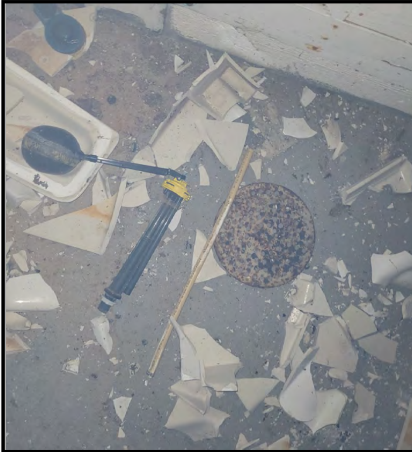
Photo 3: Building #1 bathroom floor drain.
