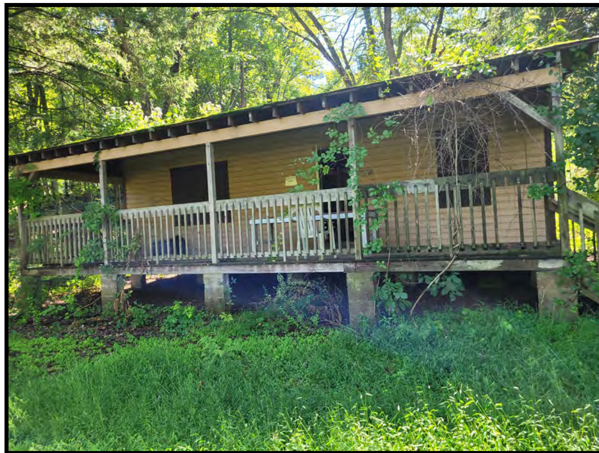
Photo 18: Building #10C exterior. Photo facing SE.
