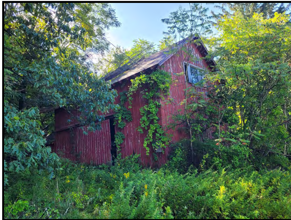
Photo 2: Building #1. Photo facing south.
