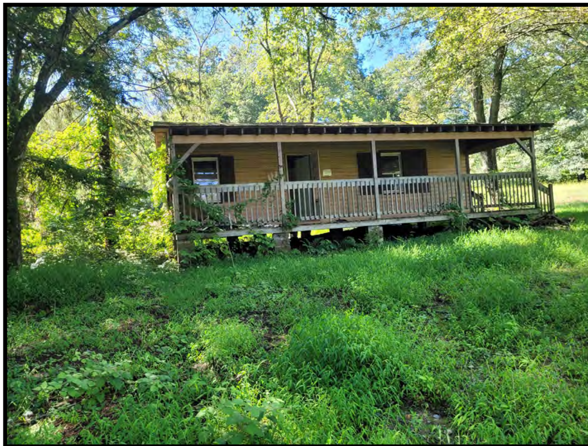
Photo 16: Building #10A exterior. Photo facing south.
