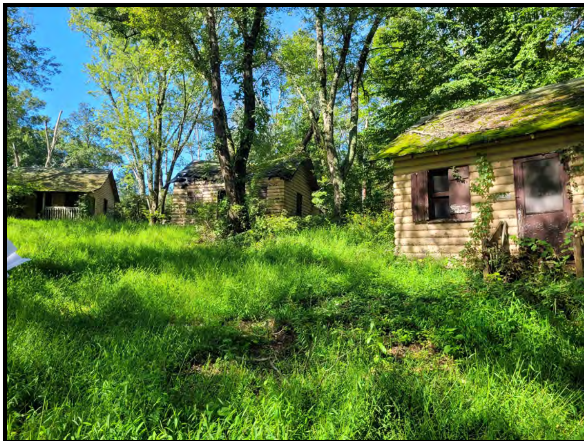
Photo 11: Buildings # 6, 7 & 8 Exterior. Photo facing west.
