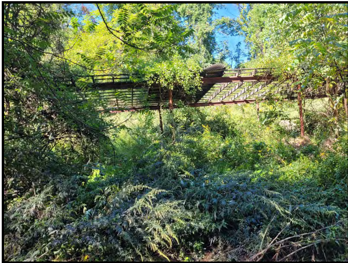
Photo 27: Building #15. Photo facing west.
