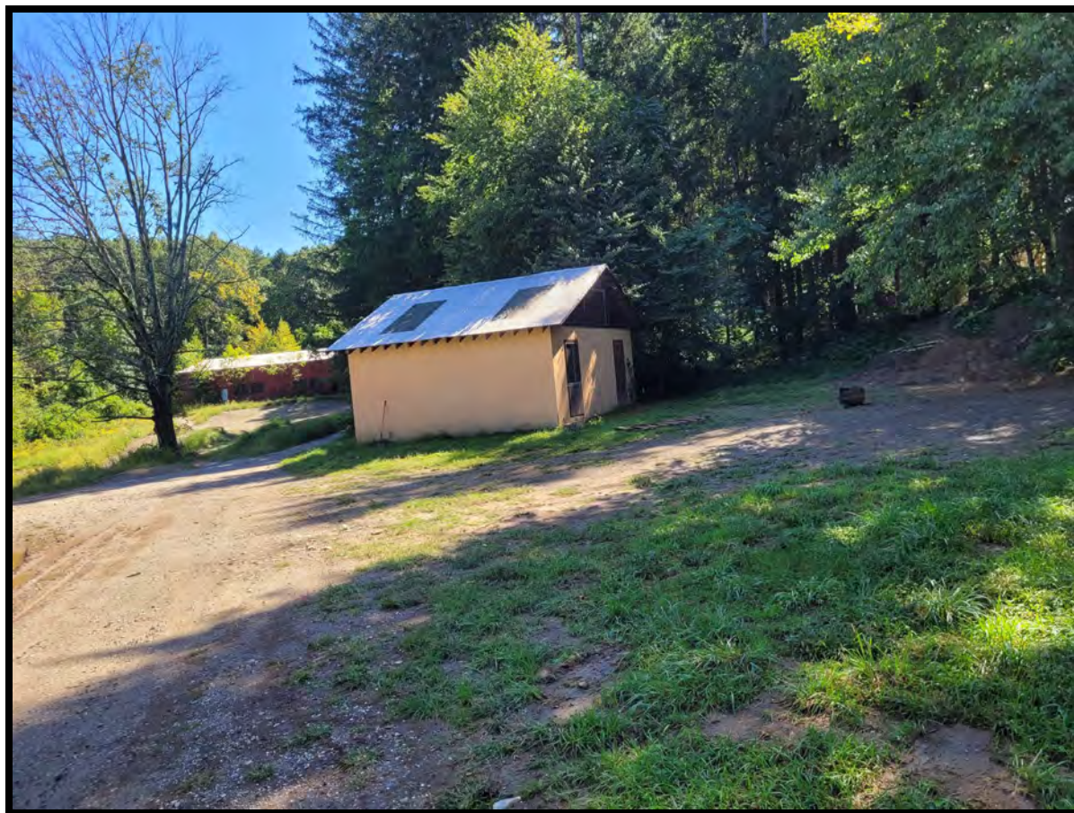
Photo 23: Building #12 exterior. Photo facing NW.
