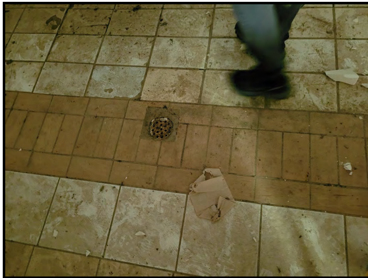
Photo 20: Bathroom floor drain in Building #11.
