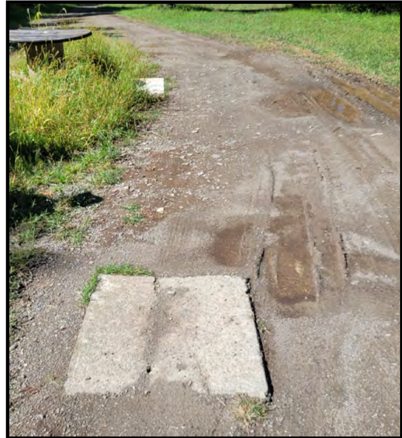
Photo 22: Presumed septic area north of Building #11. Photo facing SW.
