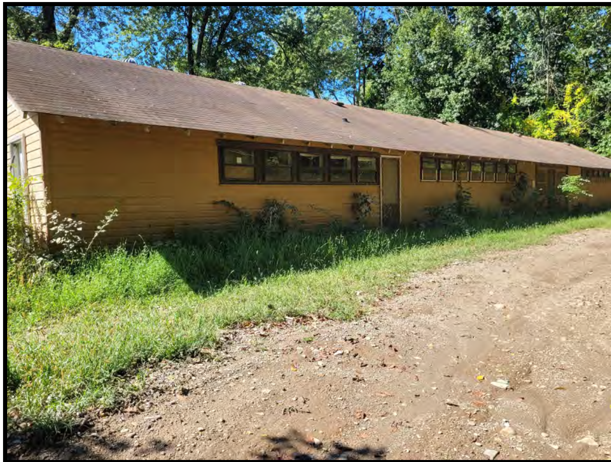
Photo 9: Building #4 Exterior. Photo facing SW.
