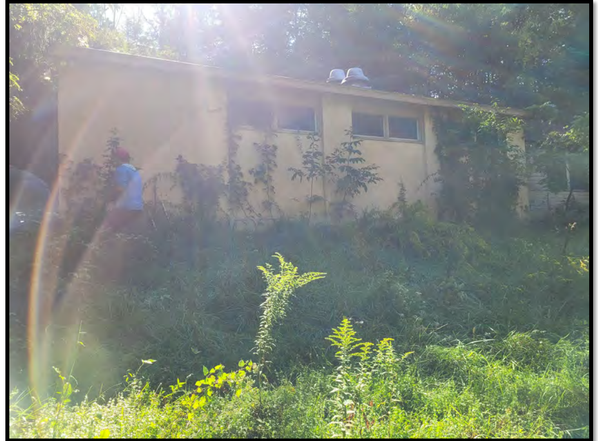
Photo 6: NW side of Building #2. Photo facing SE.
